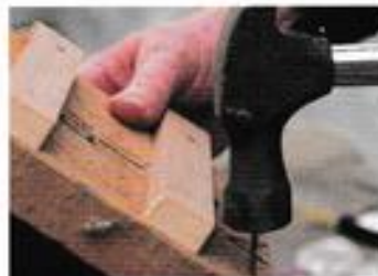
STEP 5 Using 50mm nails nail the ramp to the support.
