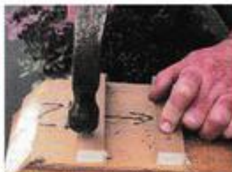
STEP 4 cut some 19mm strips from the remaining timber and nail them to the ramp to provide additional grip.
